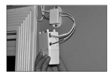
Attach the motor to the headrail.
