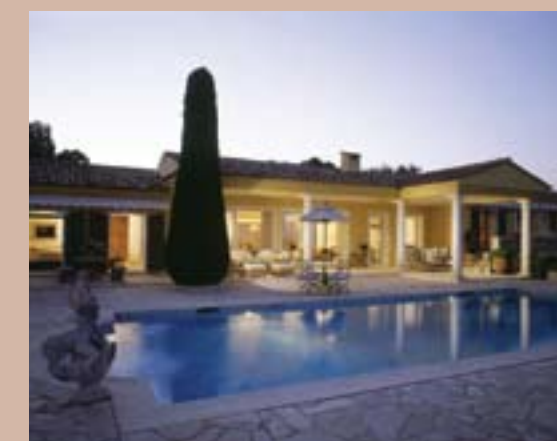
private residence, France
